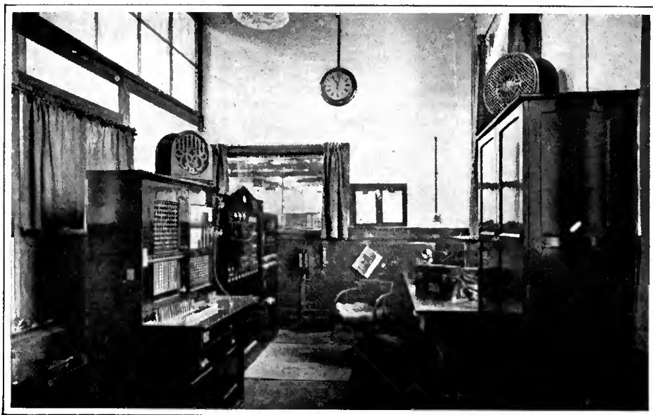
CONTROL ROOM OF 3 LO, MELBOURNE
